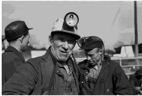
Alabama coal miners heading into the mine, ca1937. (Library of Congress)
