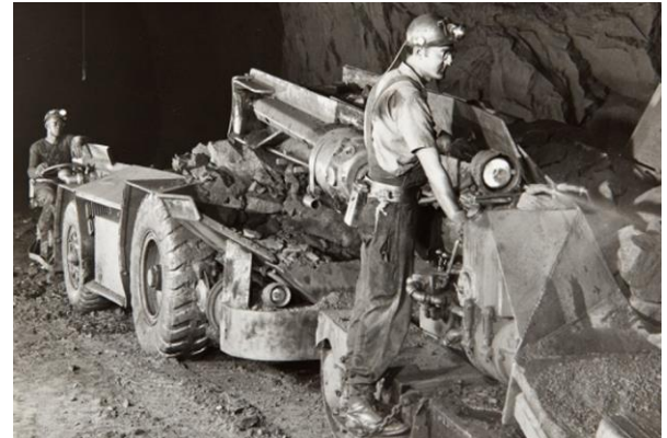
Underground mining advanced to using Joy gathering arm loaders and shuttle car haulage from slope to slope, ca1960. (Red Mountain Park)
