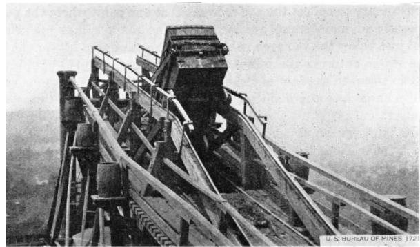
Skip at the top of the slope dumping ore into bins for loading train cars, ca1923. (USBM)
