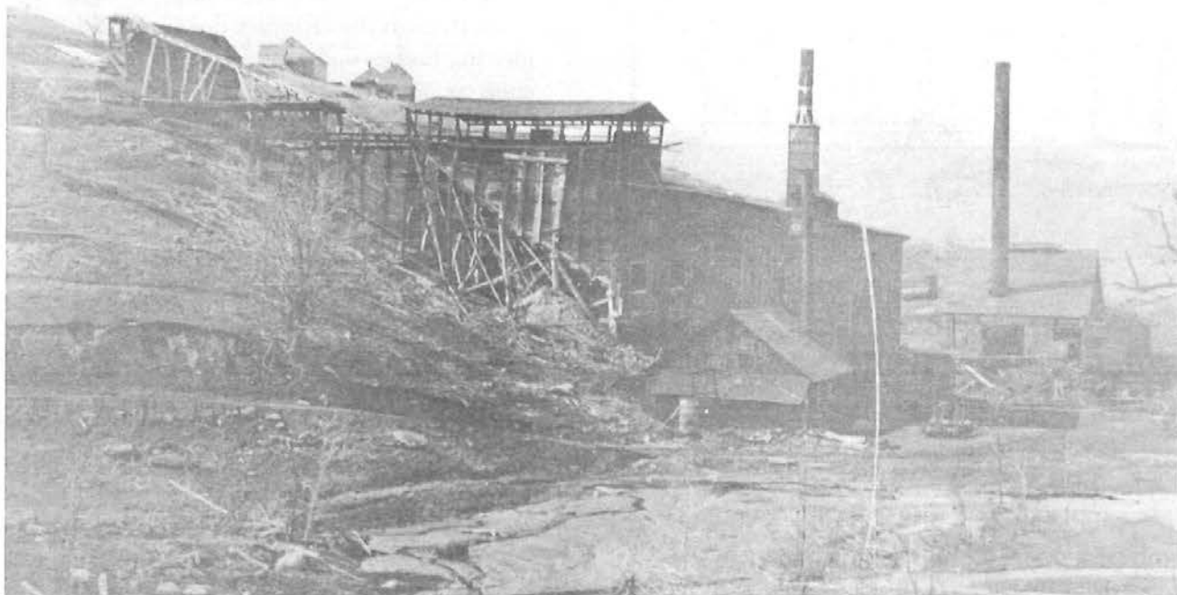
Figure 20: Idle blast and reverberatory furnaces viewed from the east. The smelter appears somewhat dilapidated, likely dating this photograph to the 1910s. The small building in front of the blast furnace with the water tank is the engine house for the blower. At the upper left lies a building believed to house matte crushing equipment, minus the stack visible in Figure 23. (Collamer Abbott Papers, University of Vermont.)
