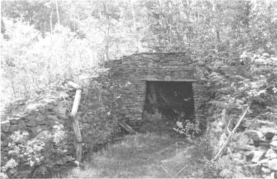
Figure 11: The Tyson Adit (1,340 feet long) was completed in 1898 and served as the mine's main entrance until final shutdown in 1958. (Photographed by the author, June, 1994.)
