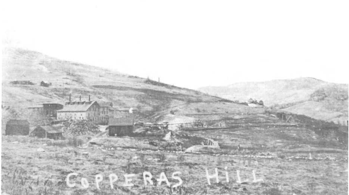
Figure 16: An overview of the Elizabeth mine complex on Copperas Hill, c. 1902. The mill buildings are left of center. Smoke from heap roasting is possibly visible near the roasting bed trestle in the center. The blast furnace is barely visible to the far right. (Courtesy of Collamer M. Abbott.)
