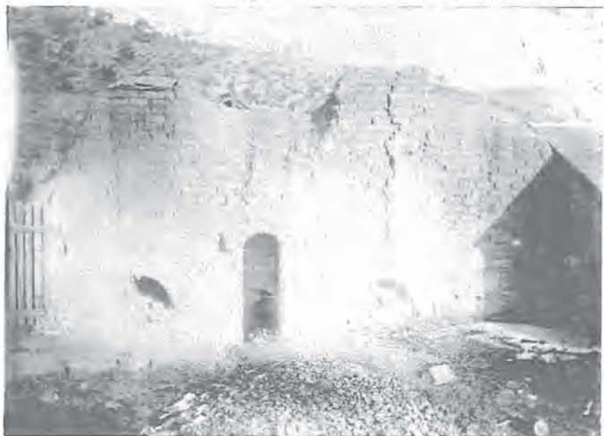
Ruins of the blast furnace built ca. 1860 by Sofio Henkle at the Hanover mine. It was similar to the works at Santa Rita. Courtesy Museum of New Mexico, Negative No. 9711.
