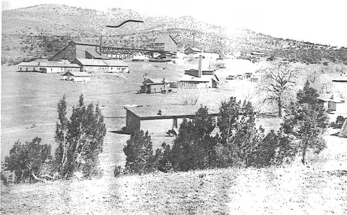
J. P. Whitney's mine hoist house and concentration mill more adapted to Michigan conditions than the Santa Rita. Hayes' smelter with tall stack sits idle below the mine. ca. 1880s. Rev. R. E. Pierce photographer, Courtesy Museum of New Mexico, Negative No. 93771 .
