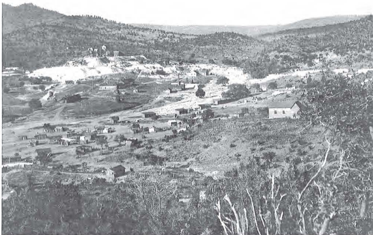
An early twentieth century view of the Santa Rita works show the smelter of Matt Hayes at center with high smokestack. To the left are the old long adobe headquarters and home of William Pierson and directly on the slope below is the lone tower remaining from the triangular fort. The view is taken from the same vantage point as Bartlett's 1851 sketch. L. C. Graton photograph ca. 1905, courtesy U. S. Geological Survey, Denver.
