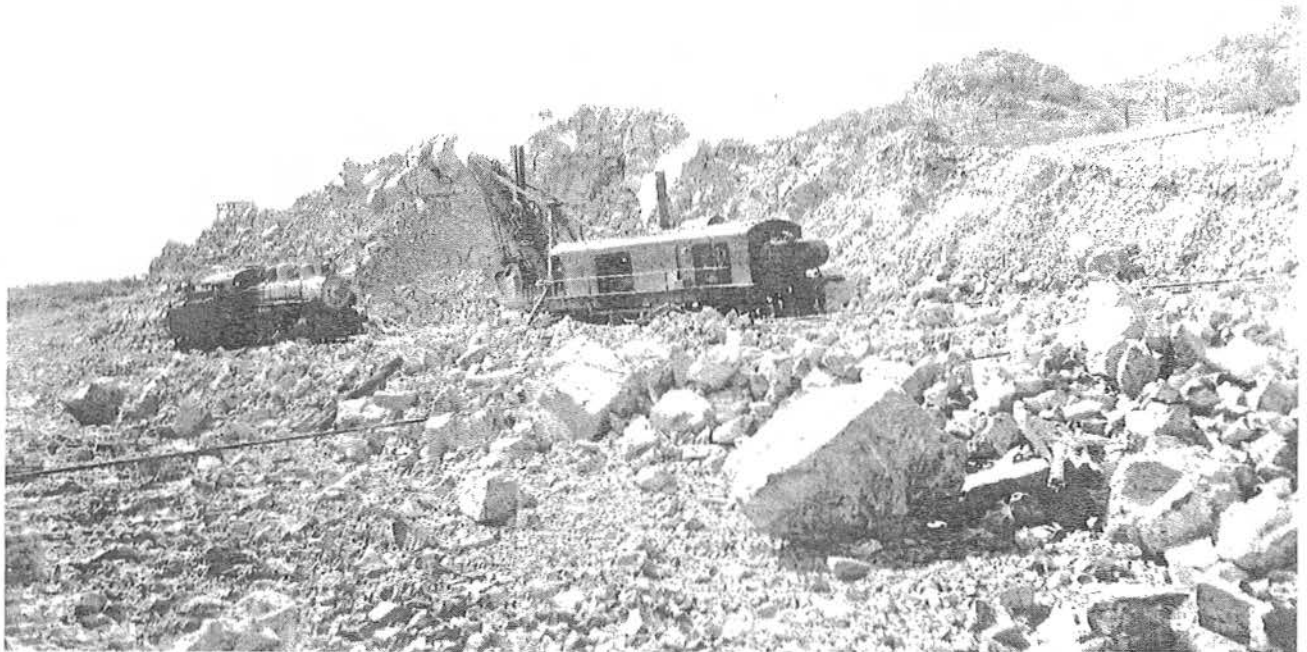
STEAM SHOVEL C. 1917. The steam shovel and rail haulage was a mining system that John C. Greenway brought with him to Ajo. Photo from George A. Newett.
