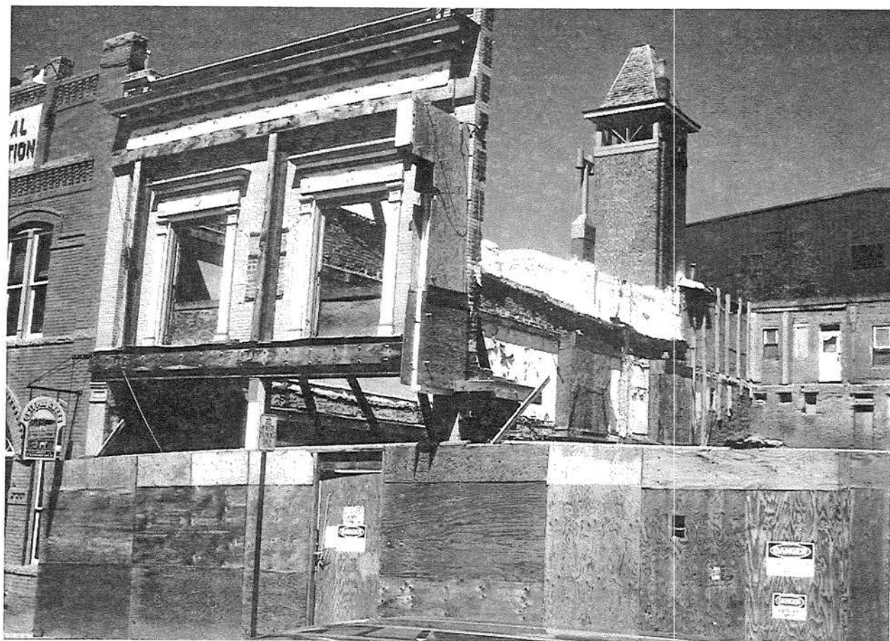
An example of what some historic preservationists call a "facadectomy." The entire building is demolished, save for the facade. The building constructed in its place retains a "historic" appearance. This facadectomy has stood thus, on Bennett Avenue in Cripple Creek, for several years. (Courtesy Eric Clements.)
