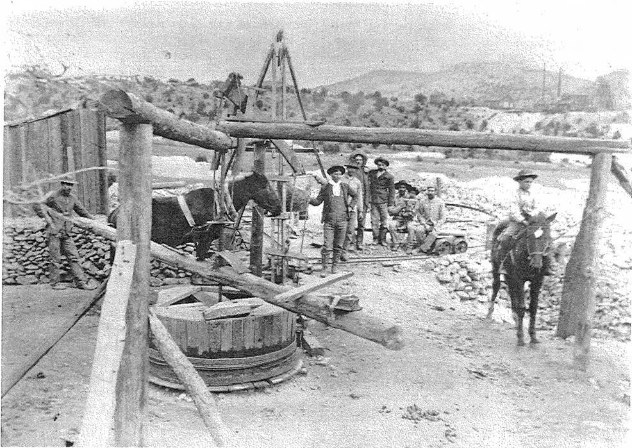
Sinking a shaft with a horse-drawn whim. This is the Ruelas lease on the Chino claim of the Chino Copper Company about 1909. (Courtesy, Benito R. Rodriguez)
