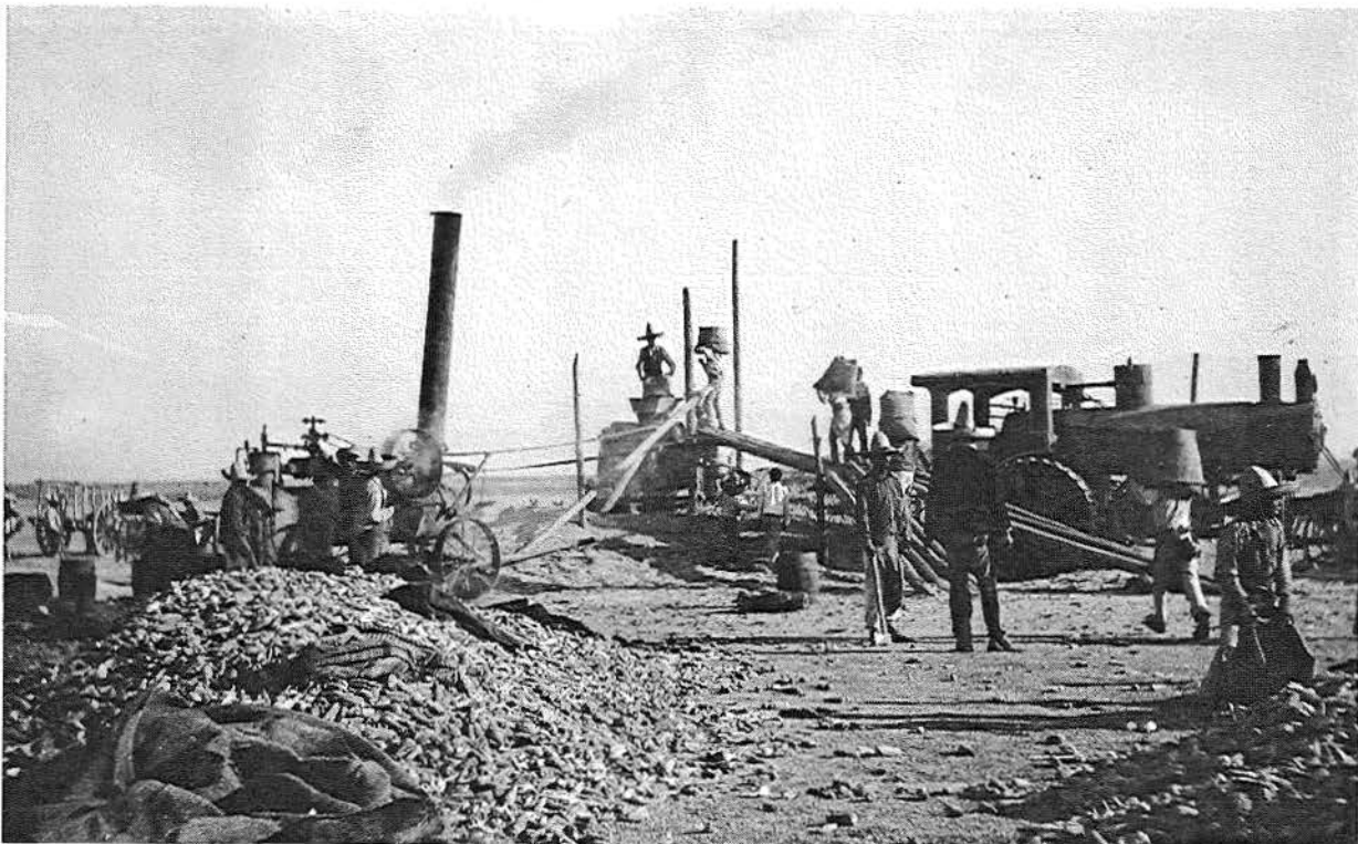
"Desgranando la Chinacates," Durango, Mexico ca. 1910. Note the corn cobs. As the corn was stripped from the dry husks the cobs were used for fuel in this mechanical adaptation to agriculture.
