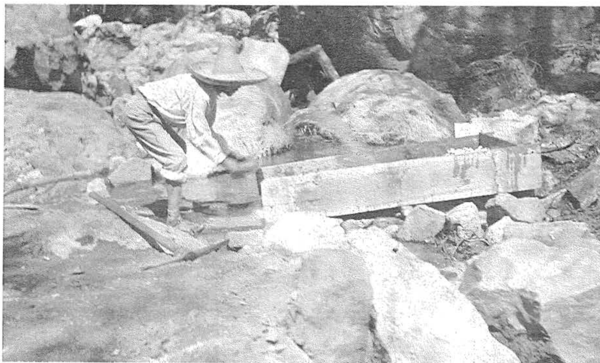
"Julio Rodriques Operating Planilla," Durango, Mexico ca. 1910. This gold miner is operating a primitive type of gold sluice on an isolated placer property.
