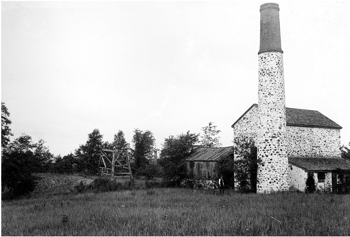
The derelict all-enclosed engine house, boiler house, and attached stack of the 24-inch rotative beam engine, first erected at the Charlestown Mine in 1852, following its removal to the Wheatley Mine in 1864. Photograph by E. B. Hardin (c. 1885), Geological Society of America, image no. 997.
