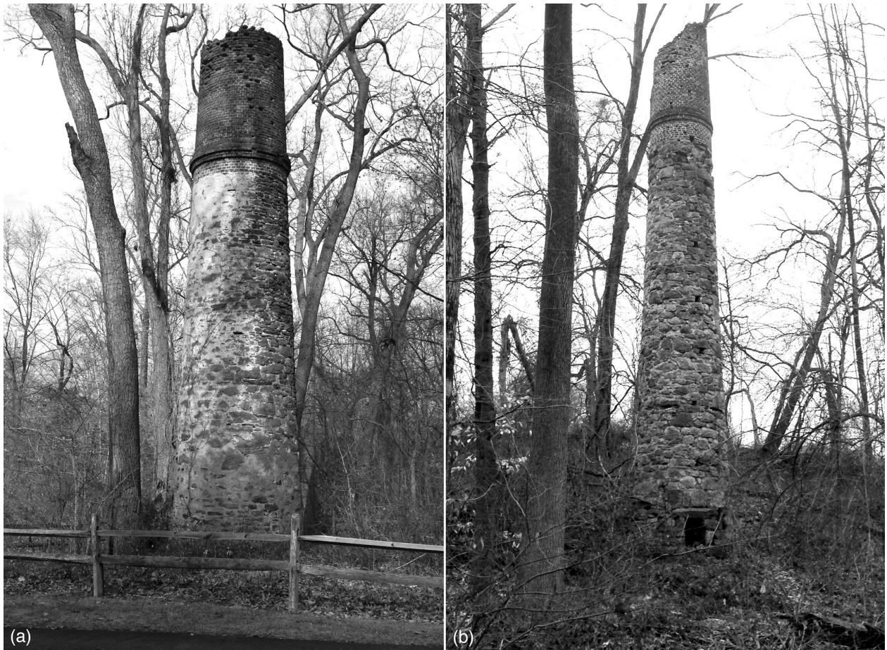
Two solitary Cornish stacks. A: The stack of the Ecton Mine's 20.5-inch, high-pressure pumping engine in the grounds of the John James Audubon Center at Mill Grove, in Audubon, Pennsylvania. The Ecton shaft lies out of the view to the right (east). B: The stack of the Brookdale Mine's 24-inch pumping engine stands beside Smith's engine shaft near Phoenixville, Pennsylvania. The flue hole at the base faced the house of the engine's single boiler.
