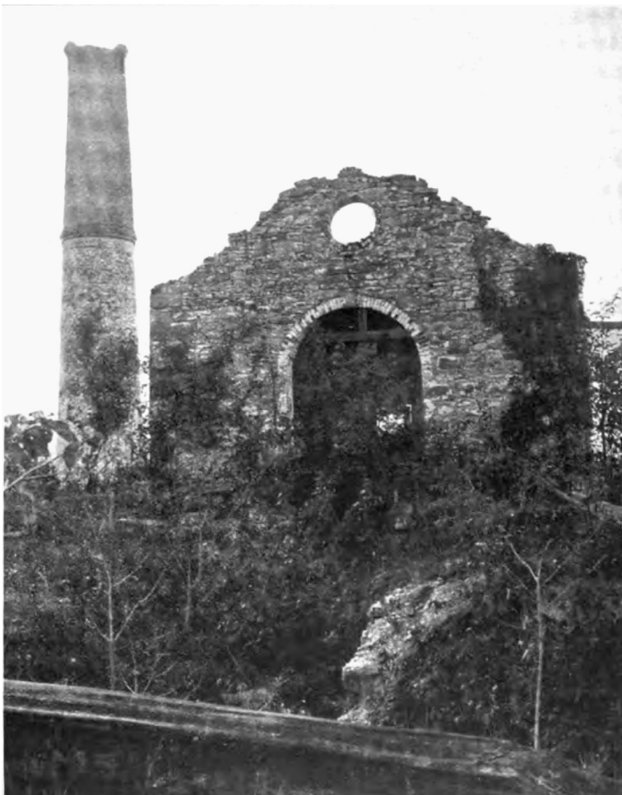
The engine house, with its large brick-arched opening, and the surviving separate stack at the Ecton mine, taken from the mouth of Ecton shaft (foreground) sometime prior to 1905. Photograph by William H. Richardson from Williams' Copper Mines at Shannonville, following p. 223.
