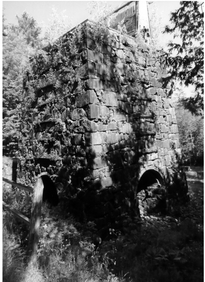
The large 1854 blast furnace at Tahawus, one of the best-preserved ruins in the historic Adirondack iron area, is still intact partly because it was little used. (Author's photo.)
