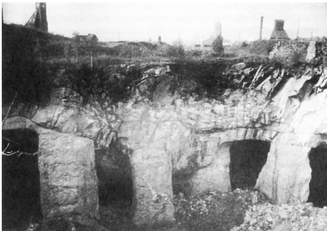
A 1915 photo of the pit in which both Witherbees, Sherman and Company and Port Henry Iron Ore Company mined iron from what were called the Old Beds. (Courtesy of the Iron Center Museum, Port Henry, from Through the Light Hole by Patrick Farrell.)
