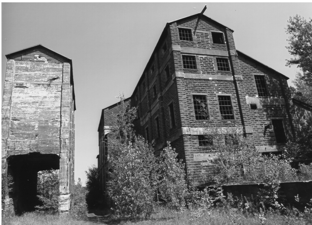
With permission, one can visit the ruins of the sintering plant (right) and sinter-loading bin for rail cars at the Chateaugay Ore and Iron Company's mill area at Lyon Mountain. (Author's photo.)
