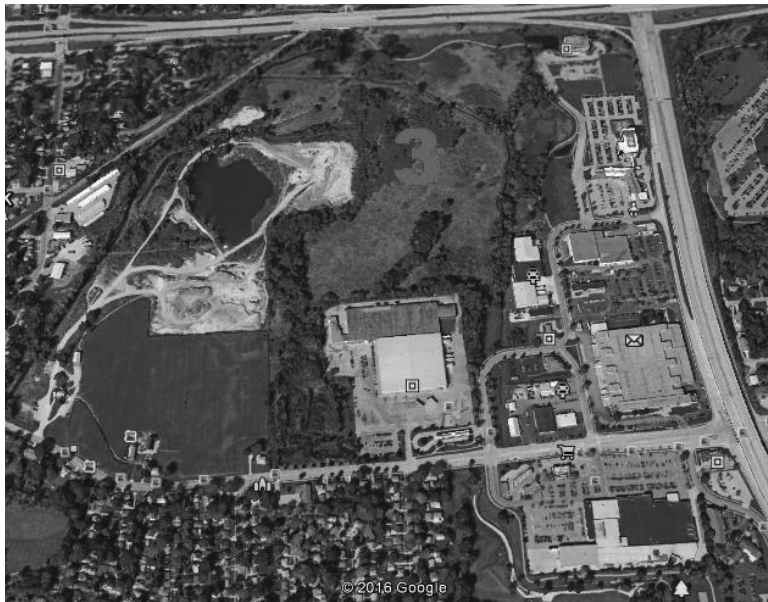
Figure 4. Quarry 3 is located north of Lake Monona and east of Lake Mendota. This quarry is surrounded mainly by a residential area and has a retention pond at its center. (Google Earth, 12 June 2014.)
