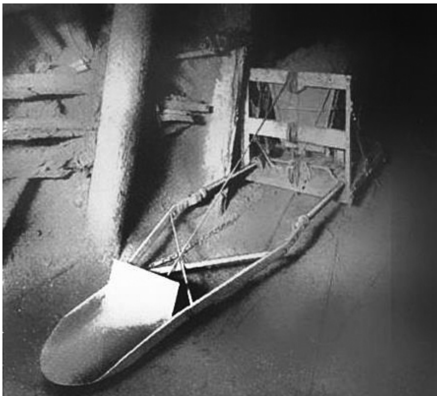
A Mayne shovel loader at Negaunee Mine in 1924. One of many types of Shovel loaders introduced across the United States between 1910 and 1925, the Mayne was designed to be as cheap and simple as possible to combat high first cost, excessive down time, high maintenance costs, and excessive space requirements – four common disadvantages of contemporary shovel-loaders. It worked effectively in soft hematite ore but proved unable to compete with the even cheaper and simpler slusher units. Pneumatic cylinders drove the shovel into the ore pile, pulled a shovel load back out, and then threw the load like a manual shoveler into the ore car shown in the background. (George R. Jackson, “The Mayne Loader,” Proceedings of the Lake Superior Mining Institute 22 (1922): 146.)
