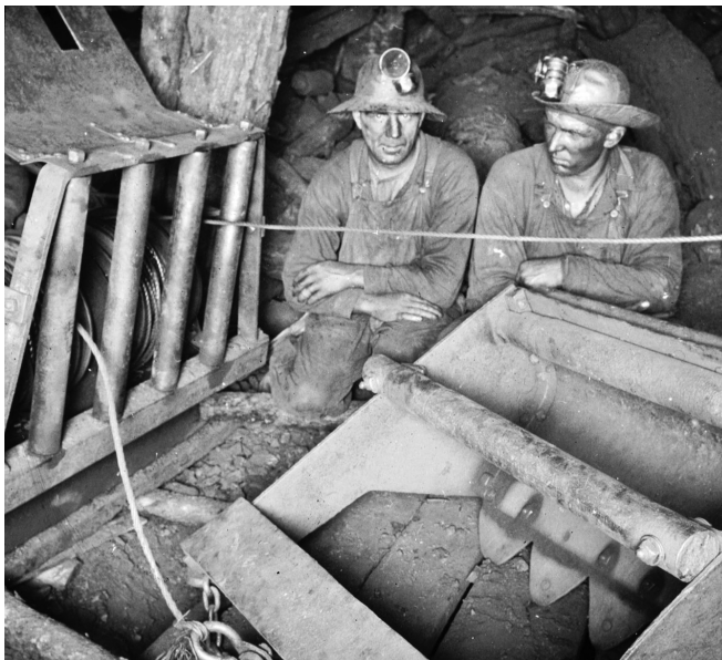
A tugger-scraper on the seventh level of Cleveland-Cliffs' Morris Mine in the 1920s. The electrically powered drum that made up the tugger part of the combination is on the left; the hoe-type scraper with teeth that the tugger's cables pulled back and forth is on the right. (Courtesy of the Michigan Tech Archives and Copper Country Historical Collections, Houghton, Michigan.)
