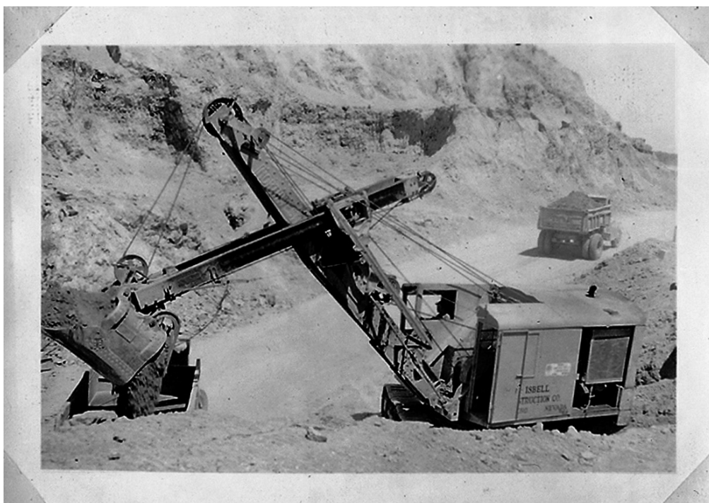
Loring initiated open-cut mining in May 1934 with a 2.5-cubic-yard shovel and a dump truck. This image shows the cut in 1937, a few months before the mine closed. (Berkley-Matthews private collection, London.)
