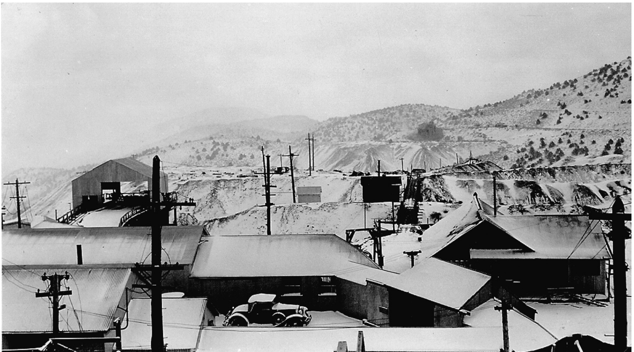
The 150-tpd flotation plant on the Hale and Norcross property west of the Fourth Ward School. (Berkley-Matthews private collection, London.)
