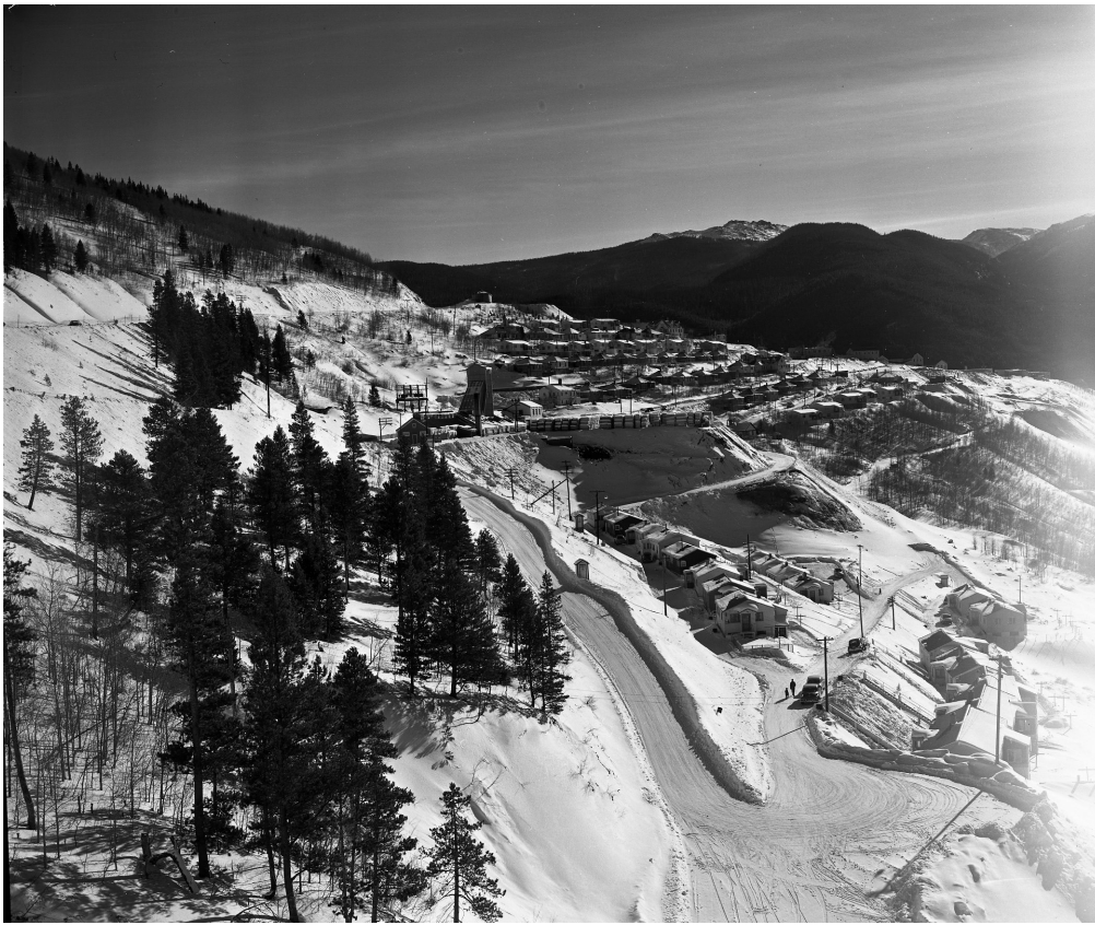
Looking down on Gilman housing. The main shaft is left of center in the photo. Stacks of mine timbers are to the right of the shaft. A small section of U.S. Highway 24 can be seen at the upper left. Photographer: Byron Stanley. (Courtesy of the Eagle County Historical Society, Eagle Valley Library District.)
