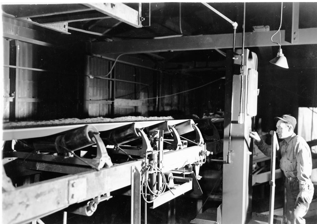
A conveyor unloading zinc from the dryer at Belden. The zinc went to the tipples to be loaded on railcars. Durbin McIlroy is monitoring the process photographed by Byron Stanley. (Courtesy of the Eagle County Historical Society, Eagle Valley Library District.)
