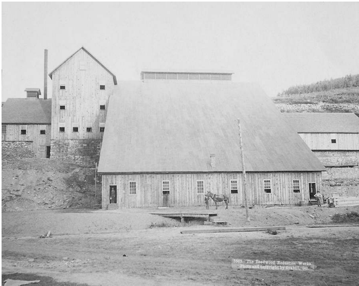
Photographer John H. C. Grabill labeled this photo "The Deadwood Reduction Works" in 1890. Because of its label, most historians believe it is of the Clark plant which burned in March 1889. More likely, it is a shot of the initial Golden Reward chlorination plant, constructed in 1889-90 by Harris Franklin. (Library of Congress, Prints and Photographs Division, John C.H. Grabill Collection, LC-DIG ppm-sc-02675.)
