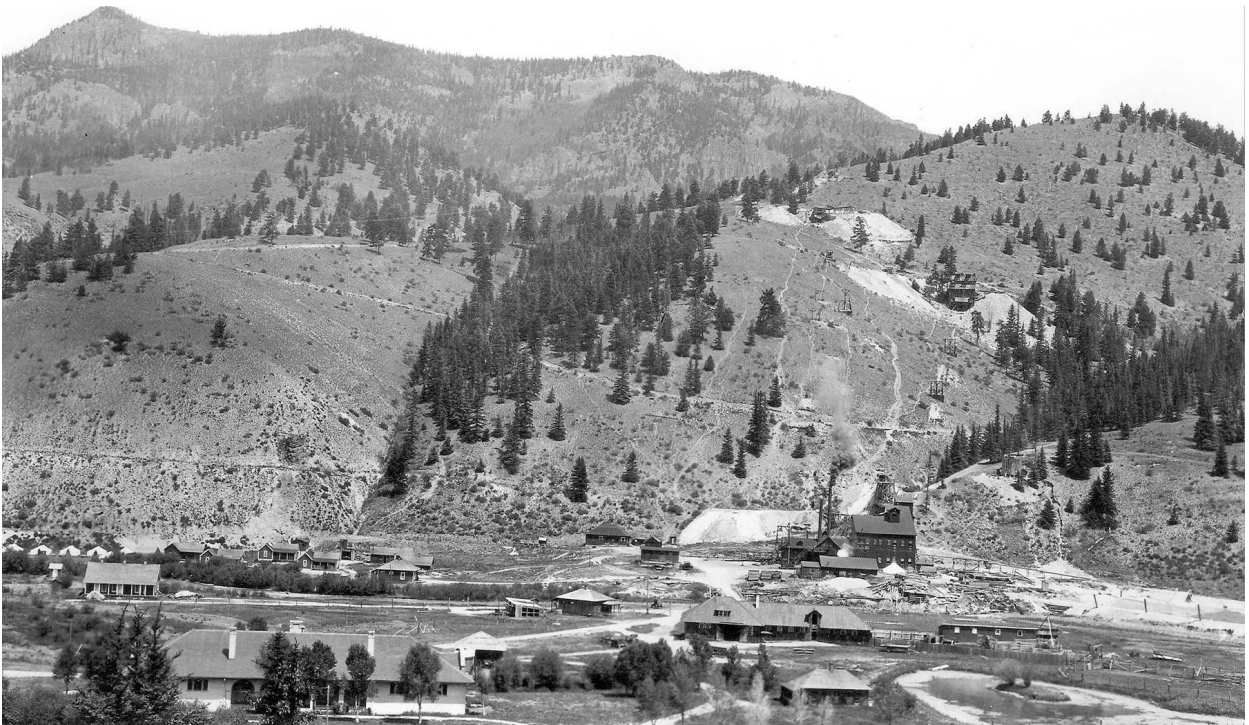
A general view of the Wagon Wheel Gap mill, dump, and camp housing, 25 July 1926. The open cut is at the crest of the mountain. The upper dump and ore bins are those of the Wilson Level. The dump, buildings, and ore bins just below the Wilson Level are those of the Intermediate Level. Aerial tram towers are visible leading from these two levels down to the mill. The buildings in the foreground belong to the 4UR Ranch and Hot Springs. (Photo EF 1325, U.S. Geological Survey Photographic Library.)
