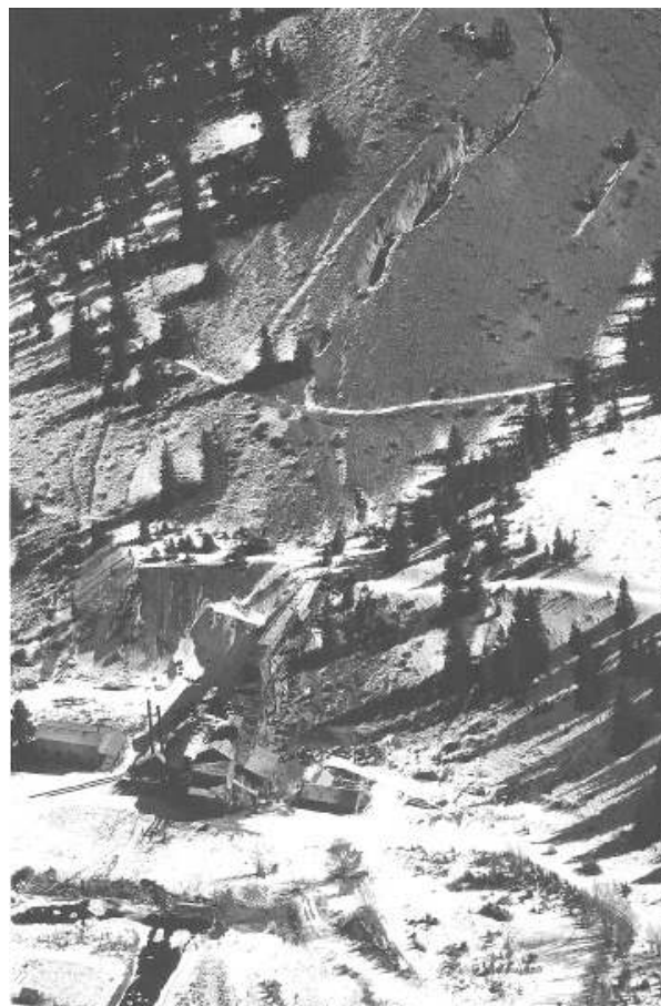
An aerial view of the Wagon Wheel Gap mill, 5 February 1999. Note the results of stoping and caving along the fluorspar vein on the hillside above the mill. (Courtesy of James G. Wark, Airphoto, Photo number 1351.)
