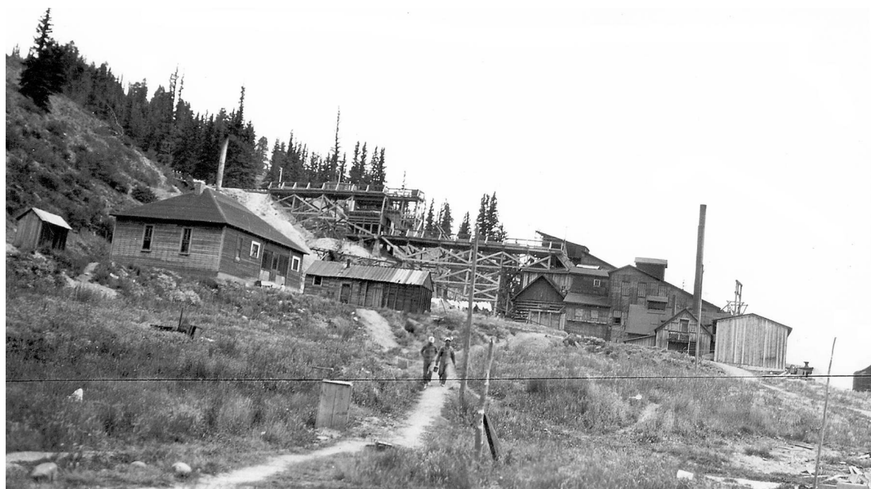
The Wagon Wheel Gap Mill, Colorado Fuel and Iron Company, 24 July 1926. (Photo EF 1324, U.S. Geological Survey Photographic Library.)
