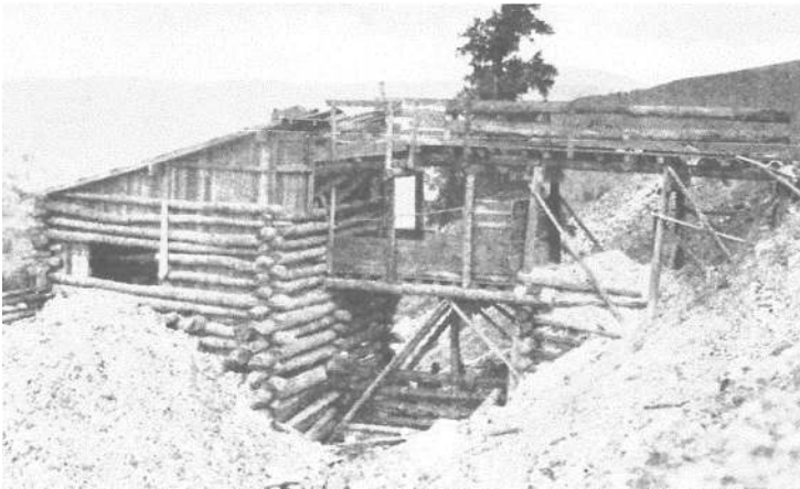
Ore bins on the Wilson Level, elevation 9,083 feet. (Aurand, “Wagon Wheel Gap District,” 65.)
