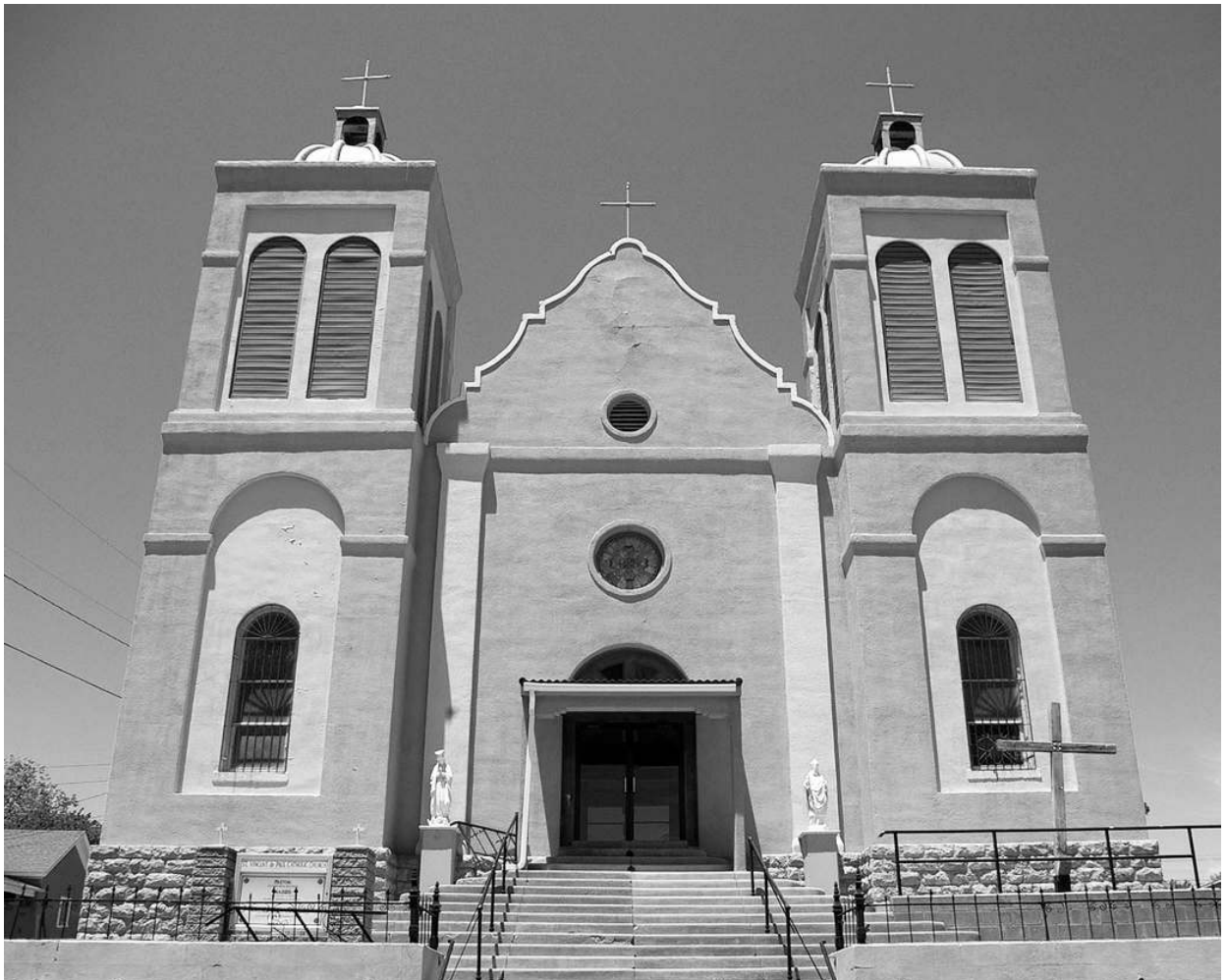
St. Vincent De Paul Catholic Church, Silver City, New Mexico. Originally constructed of stuccoed adobe between 1874 and 1876, the mission-style facade and towers were added in 1908. Throughout its history, Grant County's population has remained about 65 percent Hispanic, of whom around 90 percent are Roman Catholic.
