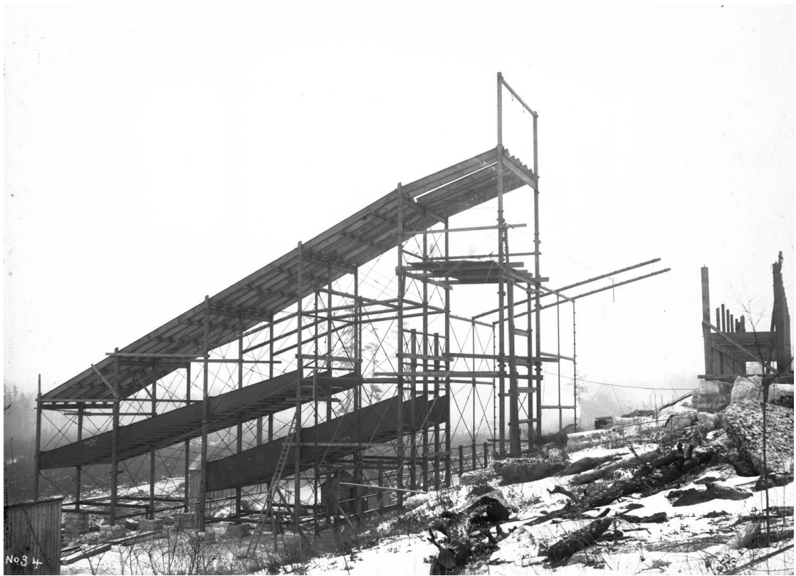
Iron breaker at Drifton, Pennsylvania, under construction about 1890. (Negative 2-8, Coxe Collection, Division of Work and Industry, National Museum of American History, Smithsonian Institution. Scanned from the glass plate negative by Eric Nystrom, 2006.)
