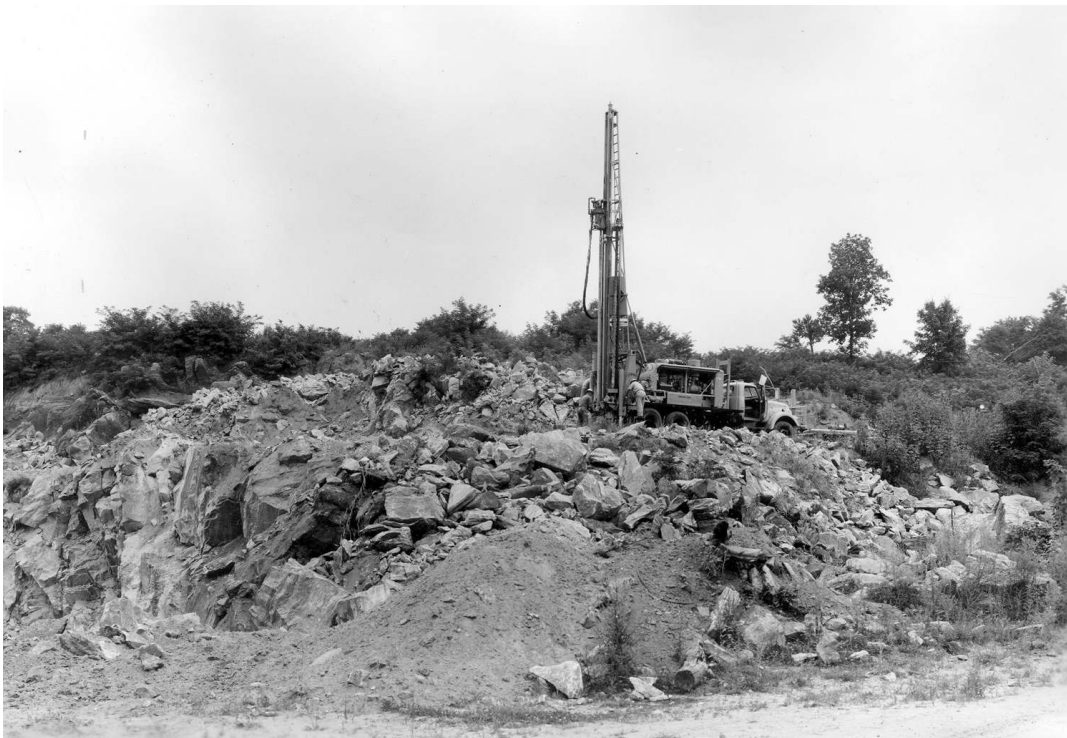
G. Edgar Harr well drilling at the Greenspring Quarry, 13 August 1956.
