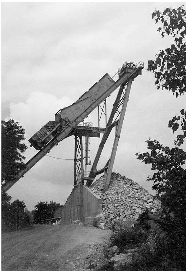
The skip car dumped twenty-six tons of shot rock every three minutes, then descended for more.
