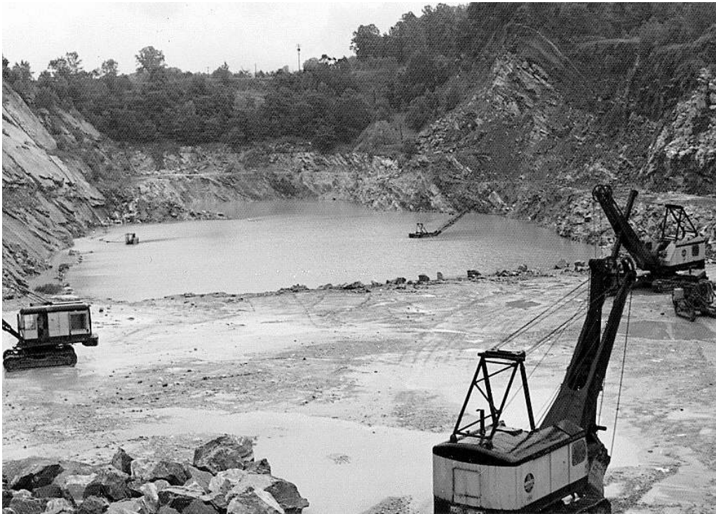
Pit flooding at Greenspring Quarry caused by Tropical Storm Agnes, 23 June 1972.
