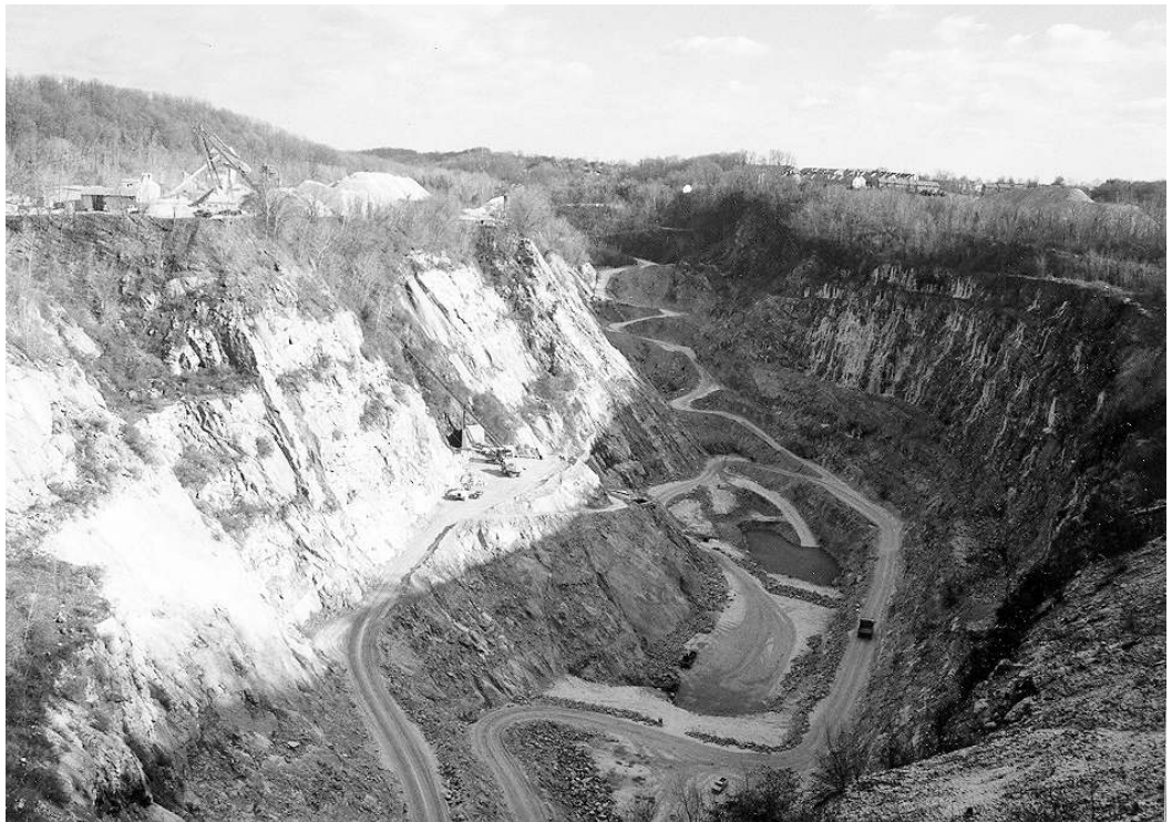
The quarry viewed from the west end, December 1999.
