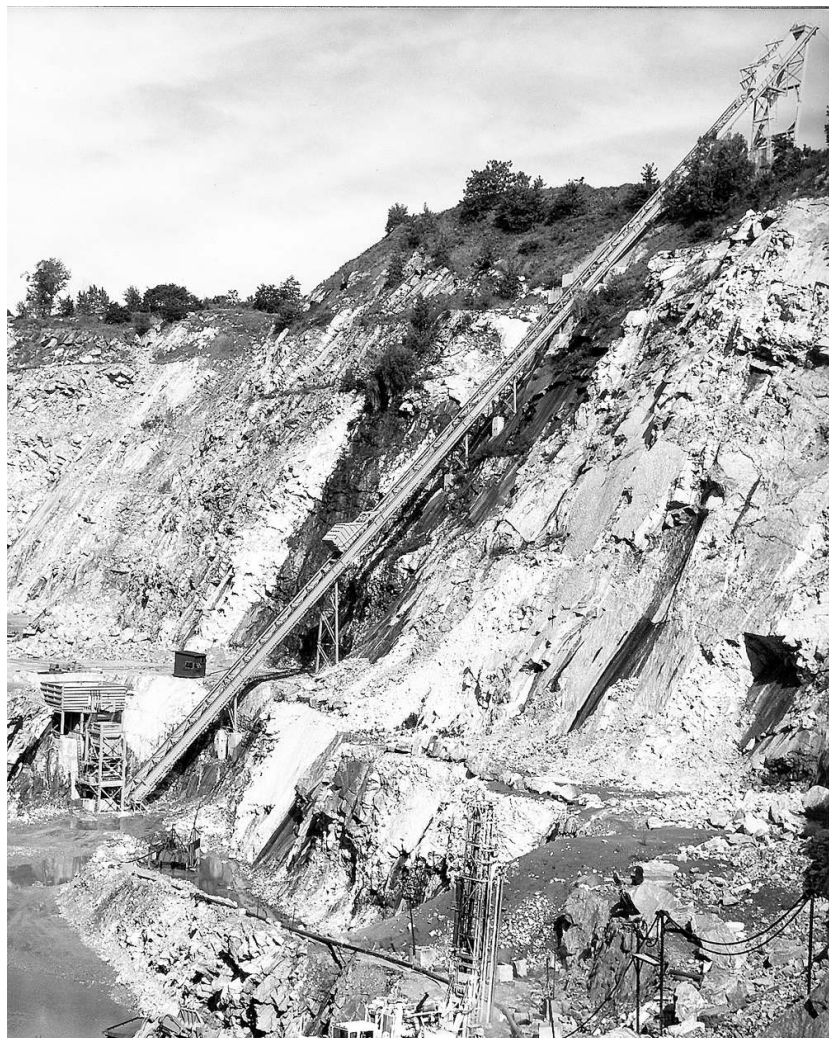
The newly installed slope hoist starting up in 1985.
