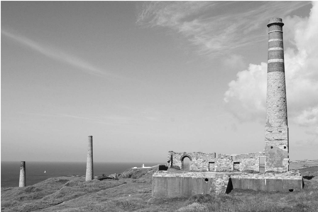
Remains of the compressor house at the Levant Mine, St. Just district. The building, built in 1901, originally contained a horizontal, triple-expansion compressor with an eighteen-foot, twenty-ton flywheel. That system was replaced by electric generators in 1919. The center chimney belonged to the stamps engine house, while the one at left was the calciner stack. Calcining furnaces roasted the Levant's tin ores to drive off arsenic, which was condensed and recovered for sale. The modern Levant dates from the 1820s, closed in 1930, and is presently owned by the National Trust. The white structure in the center distance is the Pendeen Lighthouse.
