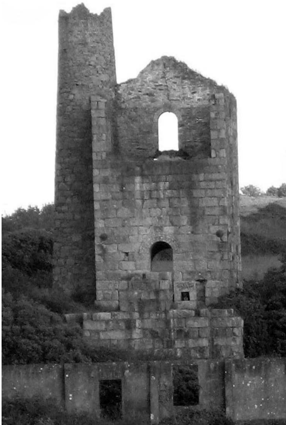
The abandoned Grenville New Stamps engine house on Carn Brea near Troon, Cornwall. The rich copper and tin lodes of Carn Brea, the eight-hundred-foot-high granite ridge rising to the south of Redruth and Camborne, made this one of the most important mining districts in the world in the eighteenth and nineteenth centuries. Built circa 1890 and finished operating about 1925, the Grenville housed an engine transferred from the nearby South Tolcarne Mine. The building is currently awaiting stabilization and is privately owned.
