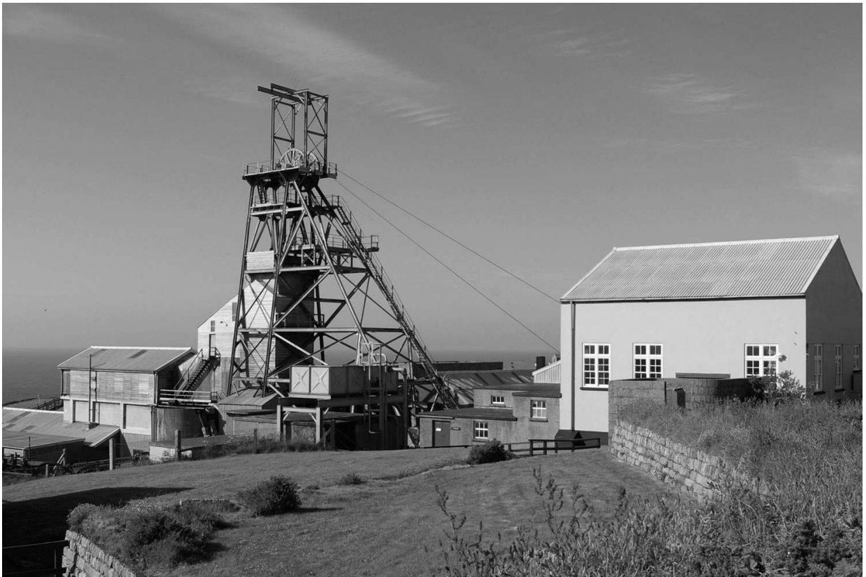
The hoist house and headframe of the Geevor Mine, St. Just district, Cornwall. Mining has occurred in the district for many centuries, but the consolidated Geevor Tin Mines Ltd. was organized in 1911. The mine ultimately occupied an area of about three square miles to a depth of 2,100 feet. The Geevor closed in 1990 and is now a museum mine preserved as part of UNESCO's Cornish Mining World Heritage Site, established in 2006.
