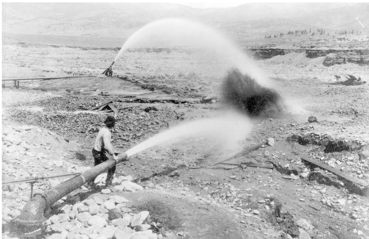
Photograph by C. W. Erdlen, taken "between 1890 and 1900," of a "miner running a hydraulic 'monitor' nozzle, Granite, Chaffee County, Colorado." (Courtesy of the Denver Public Library, Western History Collection, X-60084.)
