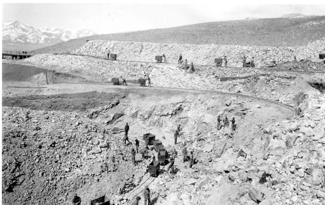
Miners loading and pushing ore cars in the Racine Boy open cut. Photograph taken by Charles E. Emery, c. 1880. (Courtesy of the Denver Public Library, Western History Collection, X-61726.)
