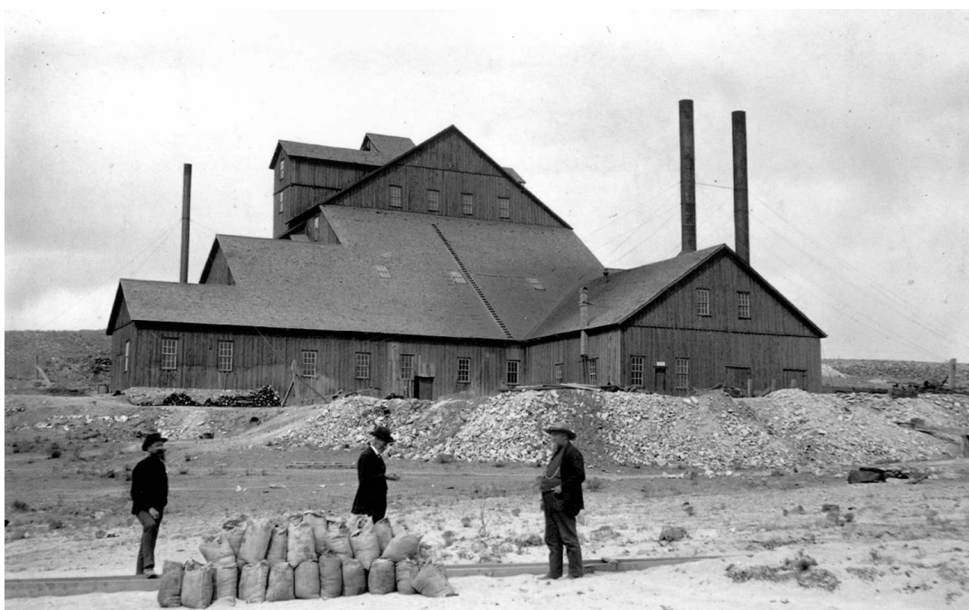
The new forty-stamp wet mill of the Silver Cliff Mining and Milling Company, completed in 1881, photographed by Charles E. Emery. (Courtesy of the Denver Public Library, Western History Collection, X-60785.)
