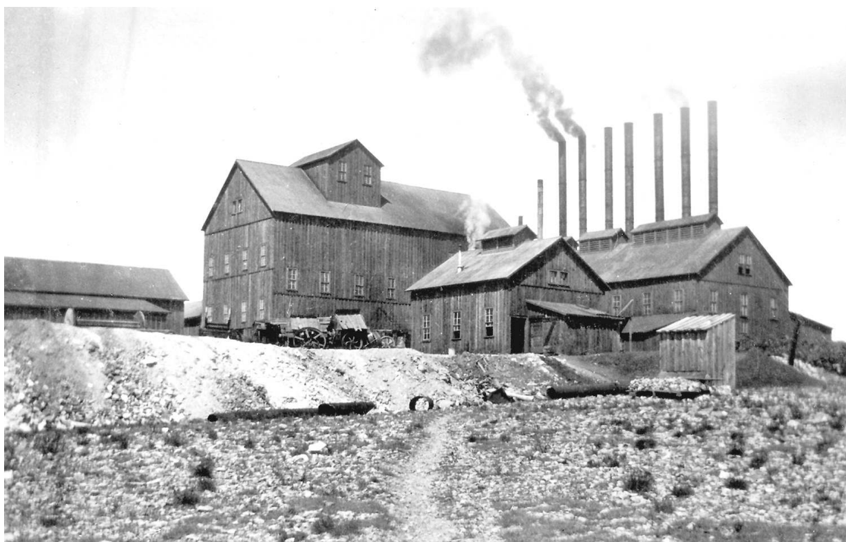
The Geyser Shaft's surface plant. The shaft house is the large building in the center of a photo taken c. 1896. (Courtesy of the Denver Public Library, Western History Collection, C-61723.)
