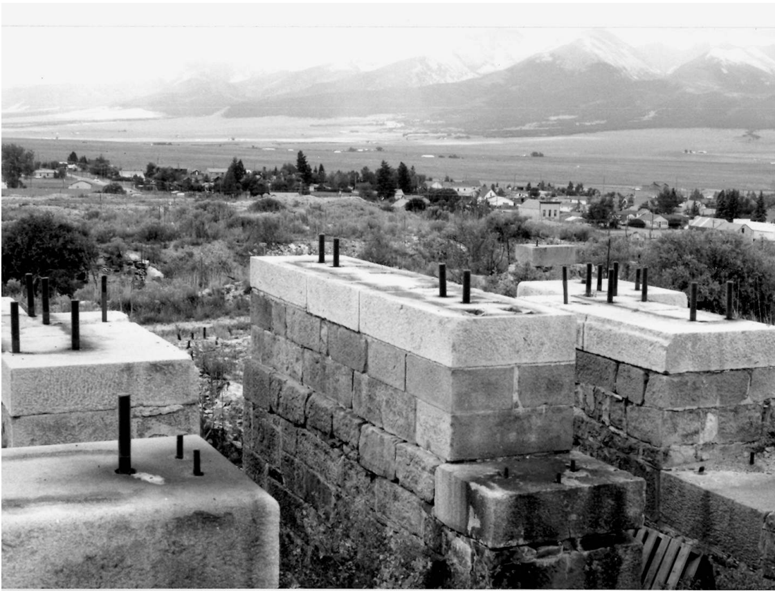
The stone foundations for the Geyser Shaft's double-reel flat-rope hoist, looking south, with Silver Cliff and the Sangre de Cristo Mountains in the background, August 2000. (Author's photo.)
