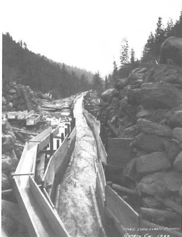
Wooden flumes, 1933. The first two sections of the flumes were lined with small lodgepole pine logs that served as riffles. (Courtesy of Arnold G. Holding.)
