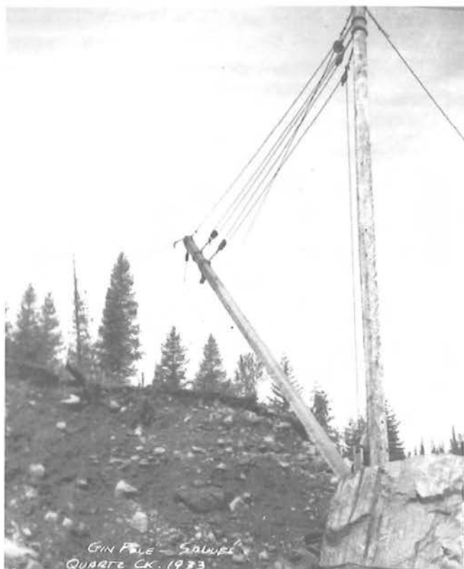
The hand-built pole hoist, dubbed the gin pole, used to move large rocks, 1933. (Courtesy of Arnold G. Holding.)
