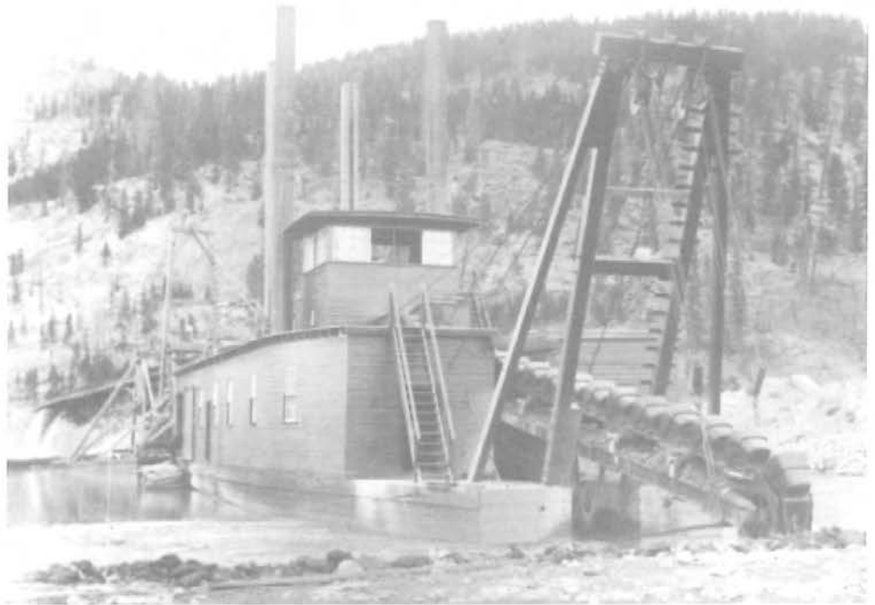
View of the Bucyrus Dredge, showing the bucket line. (Courtesy of the Colorado Historical Society.)
