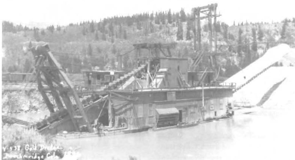
The Tonopah No. 1 Dredge on the Blue River. Note that the stacker is covered by canvas, allowing winter operation. (Authors' collection.)
