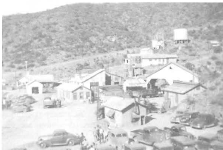
The Borianana mining camp in 1937, about the time of the transfer of the property from Sievers family-run Borianana Mining and Milling Company to the Molybdenum Corporation of America. (Courtesy of the Mohave County Museum of Art and History.)
